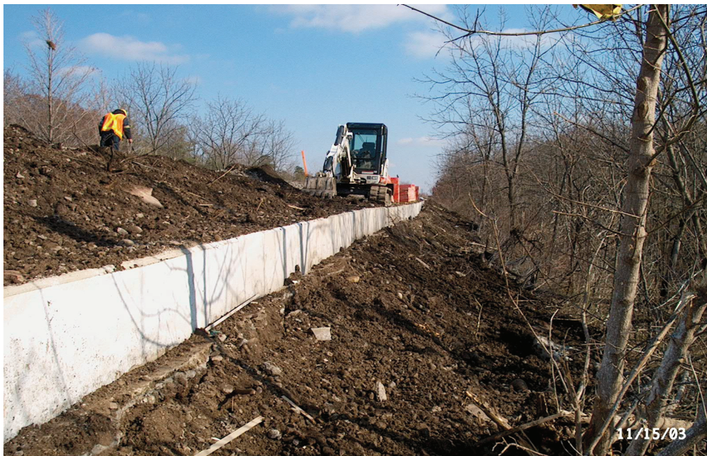
Figure 8. Embankment grading following pile cap installation.
