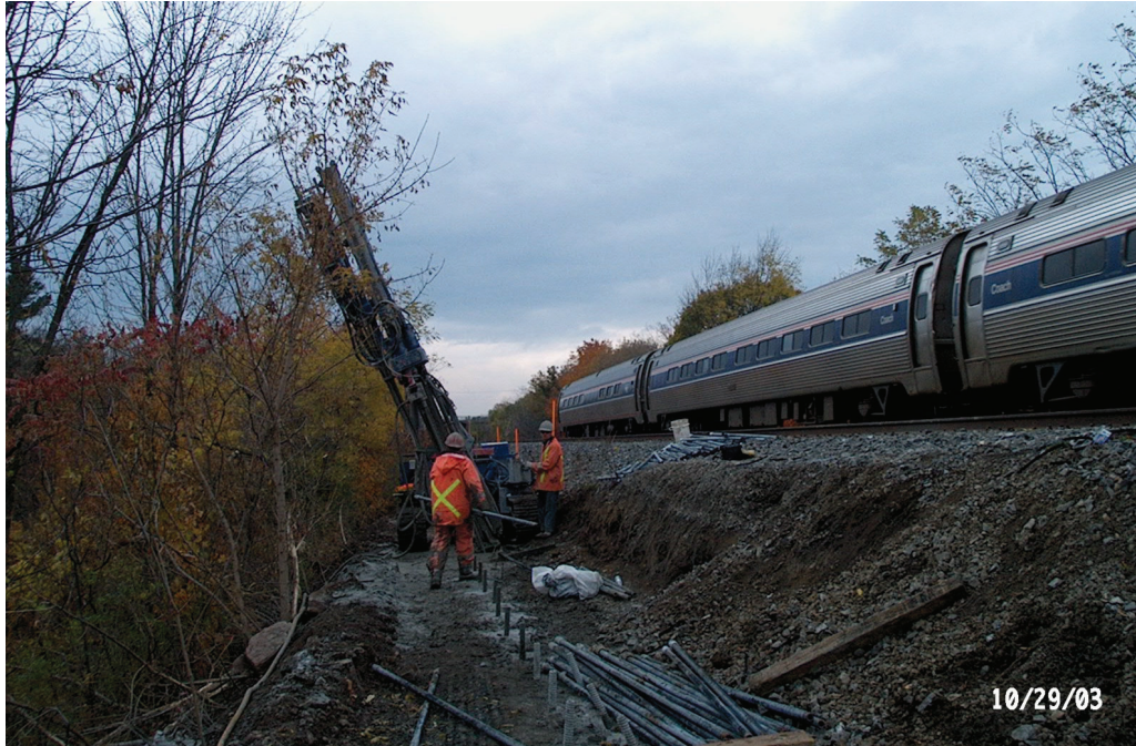
Figure 7. Installation of micropiles during track operation.
