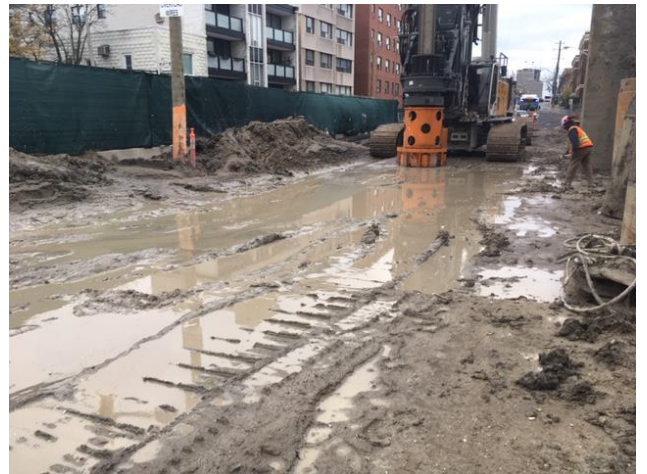
Fig 7: Example of a poorly prepared platform with poor drainage
