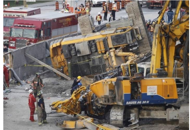
Fig 5: Lack of adequate platform results in damage to adjacent property
