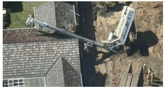
Fig 5: Lack of adequate platform results in damage to adjacent property
