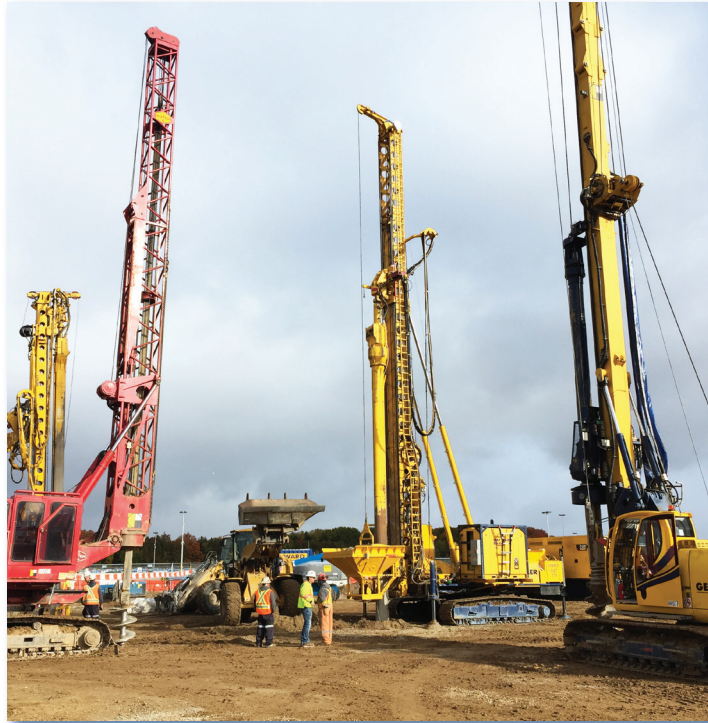
Keller aggregate pier and pre-drill equipment.
