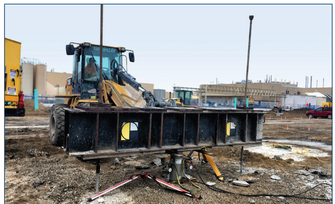
Aggregate pier modulus test to verify system performance.
